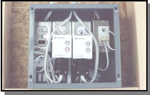
BEFORE (during construction)
